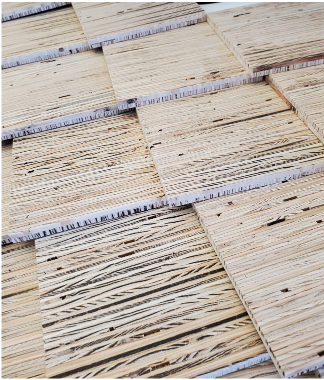
Figure 6. Plywood Crosslam in a fishscale façade. Author.
